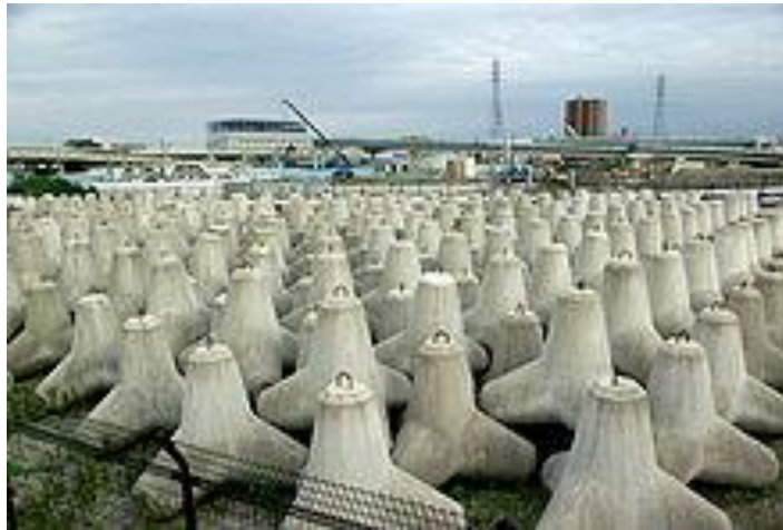
Figure 9. Tetrapods one variety of structures used to stabilize beaches.
