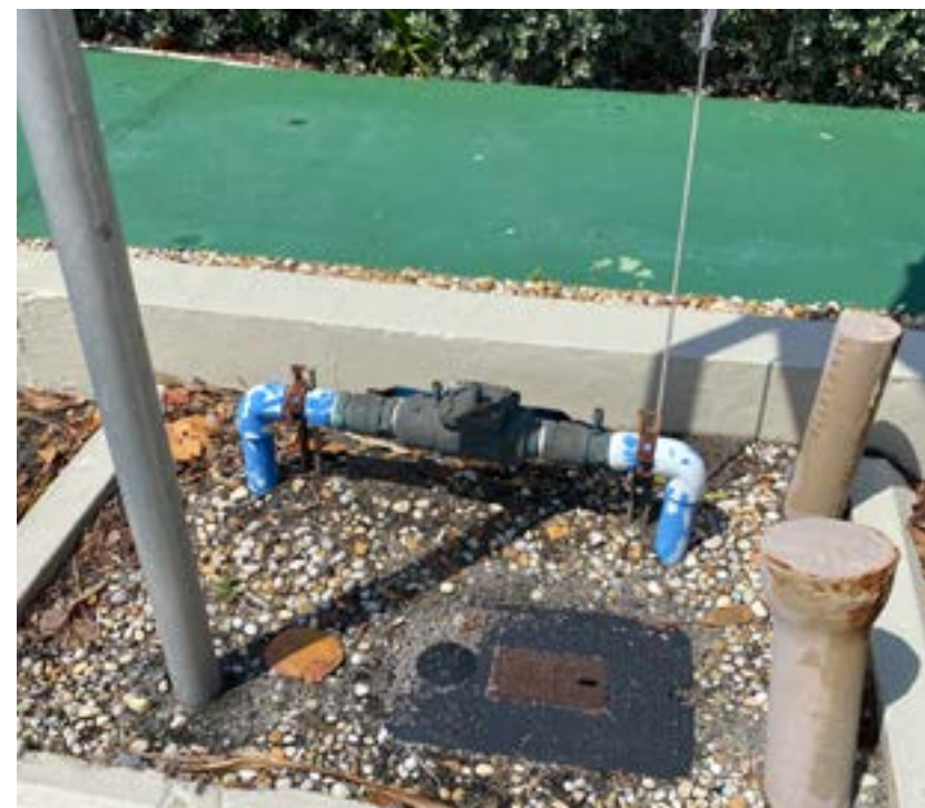
Along A1A- Utilities
