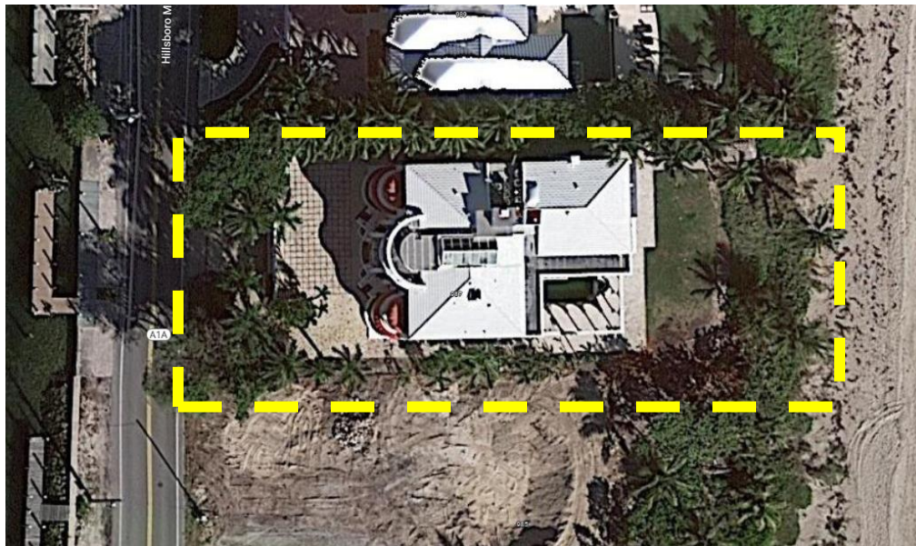
987 Hillsboro Mile – Location of proposed renovations and addition
