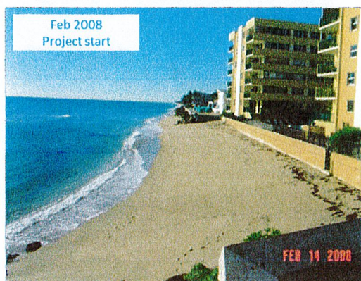
Fig. 10 – Project start at R6.5 looking south
