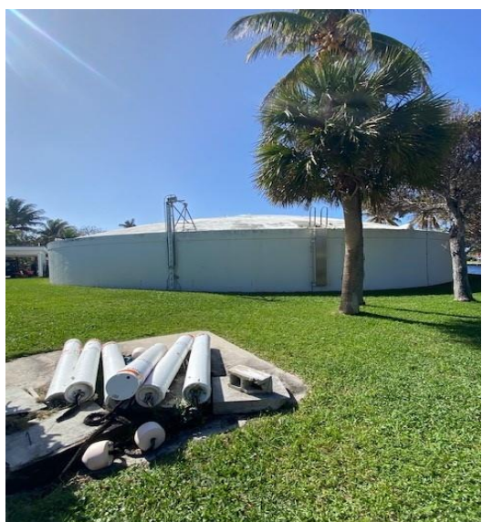
Beach Repump Station GST
