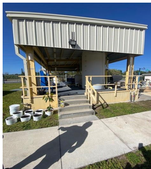
Treatment Chemical Storage
