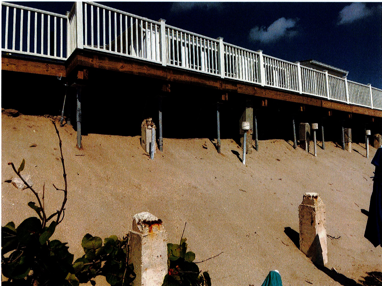
Photo 1. View of the temporary shoring underneath the walkway and cut piles in the foreground.
