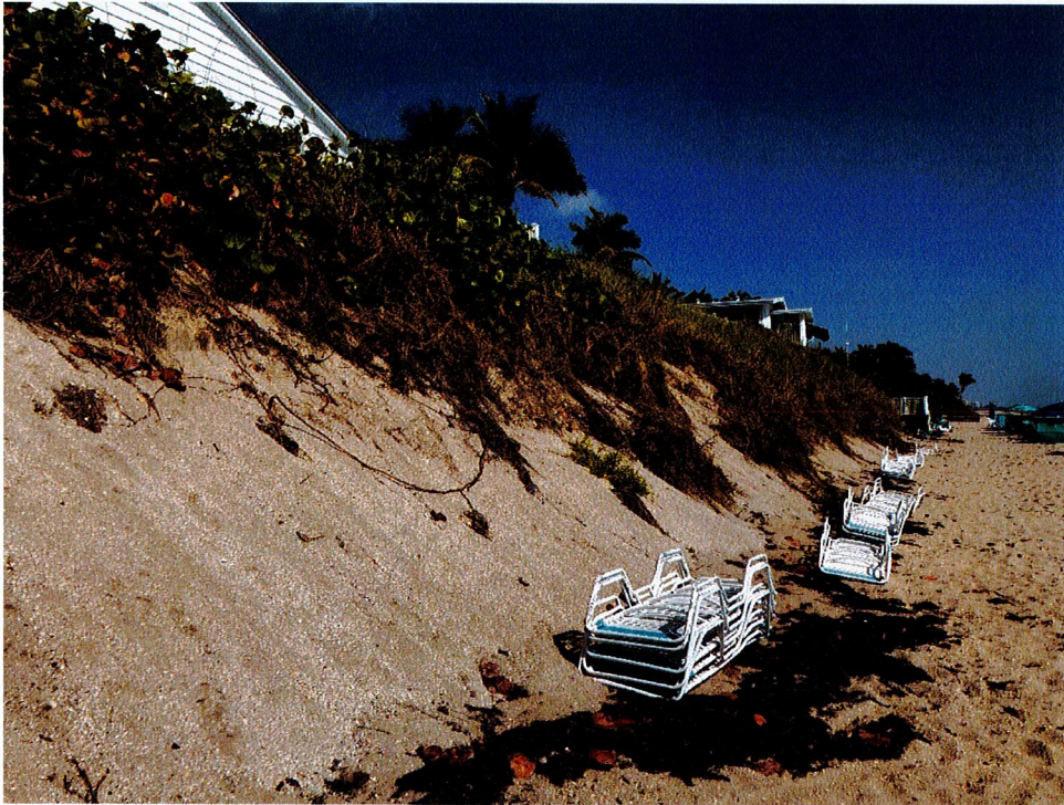
Photo 2. Denuded section of dune due to wave action and undercutting of the dune.
